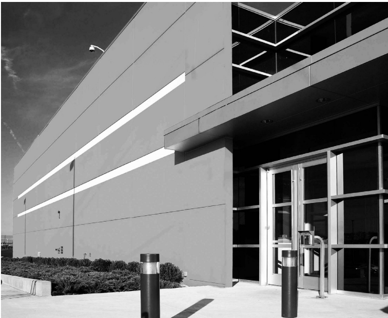
ACC4, located in Ashburn, VA
