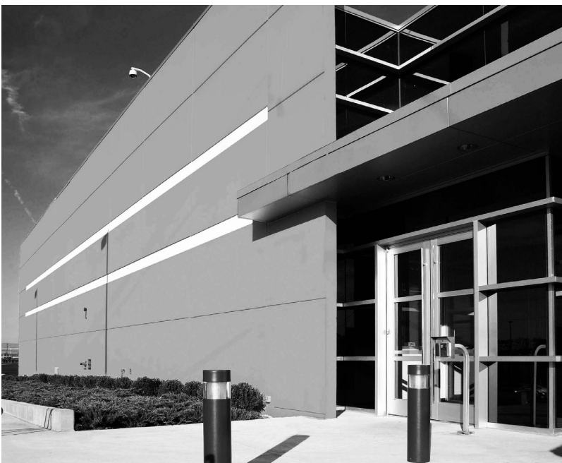
ACC4, located in Ashburn, VA
