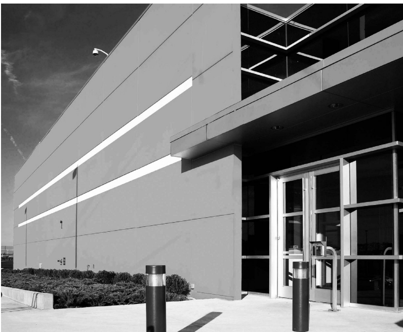
ACC4, located in Ashburn, VA
